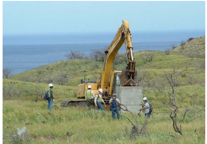
A crane carries an aluminum blast shield that is used around potentially unstable unexploded ordnance to protect area homes. Courtesy Photo.
