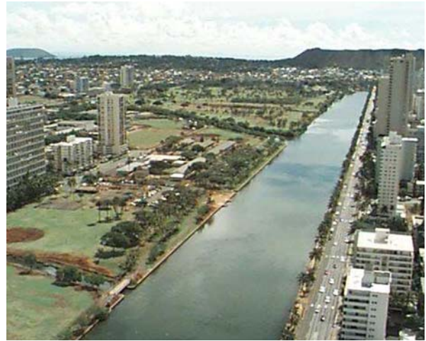
The Ala Wai Canal, a historical landmark in Waikiki, is plagued with a variety of modern day ailments which could affect its ability to prevent major flooding. USACE Photo.
